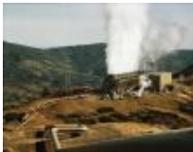
**Geothermal** - Heat from the Earth's core can also be used to generate electricity. This geothermal energy (hot water and steam) is channeled through pipes to drive turbines - connected to generators, which produce the electricity.
