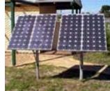
**Sunlight** - Solar cells (made from silicon) enable the energy from the sun to be transformed (photoelectric effect) into electricity.
