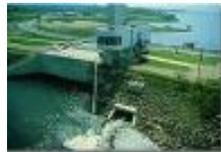
**Tides** - moving water can power turbines, which then run generators. When the tide comes in, the water is trapped in large reservoirs and then allowed to flow out past turbines.
