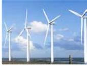
**Wind** - this energy is harnessed by large propeller-type blades, which turn a shaft - connected to a generator.
